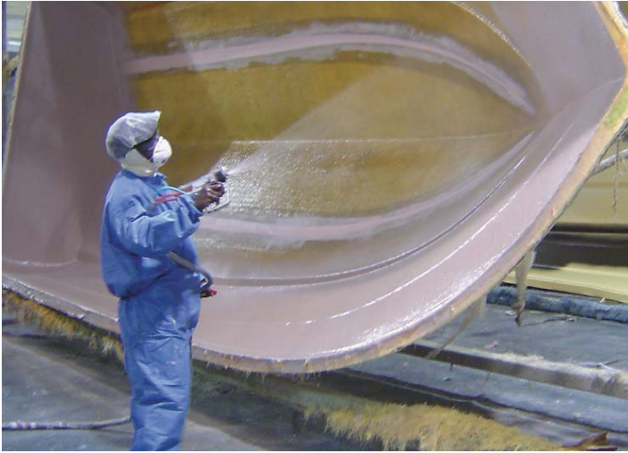
Sprayable application of SprayCore 2000-OS Coring Material
